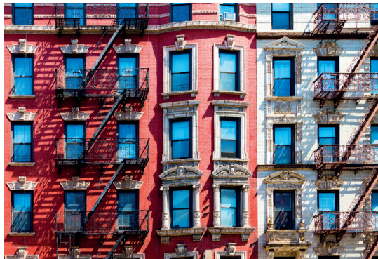
apartment building bloque de pisos
