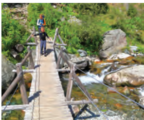
3 over the bridge
